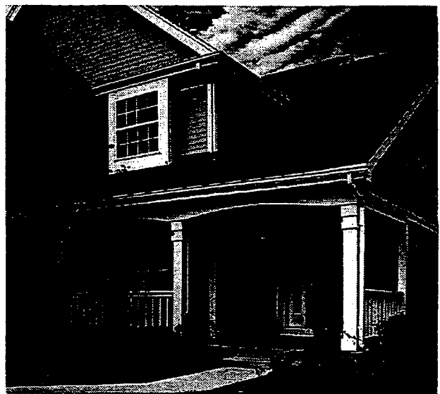
Porch Entry & Second Floor Bay Projection
